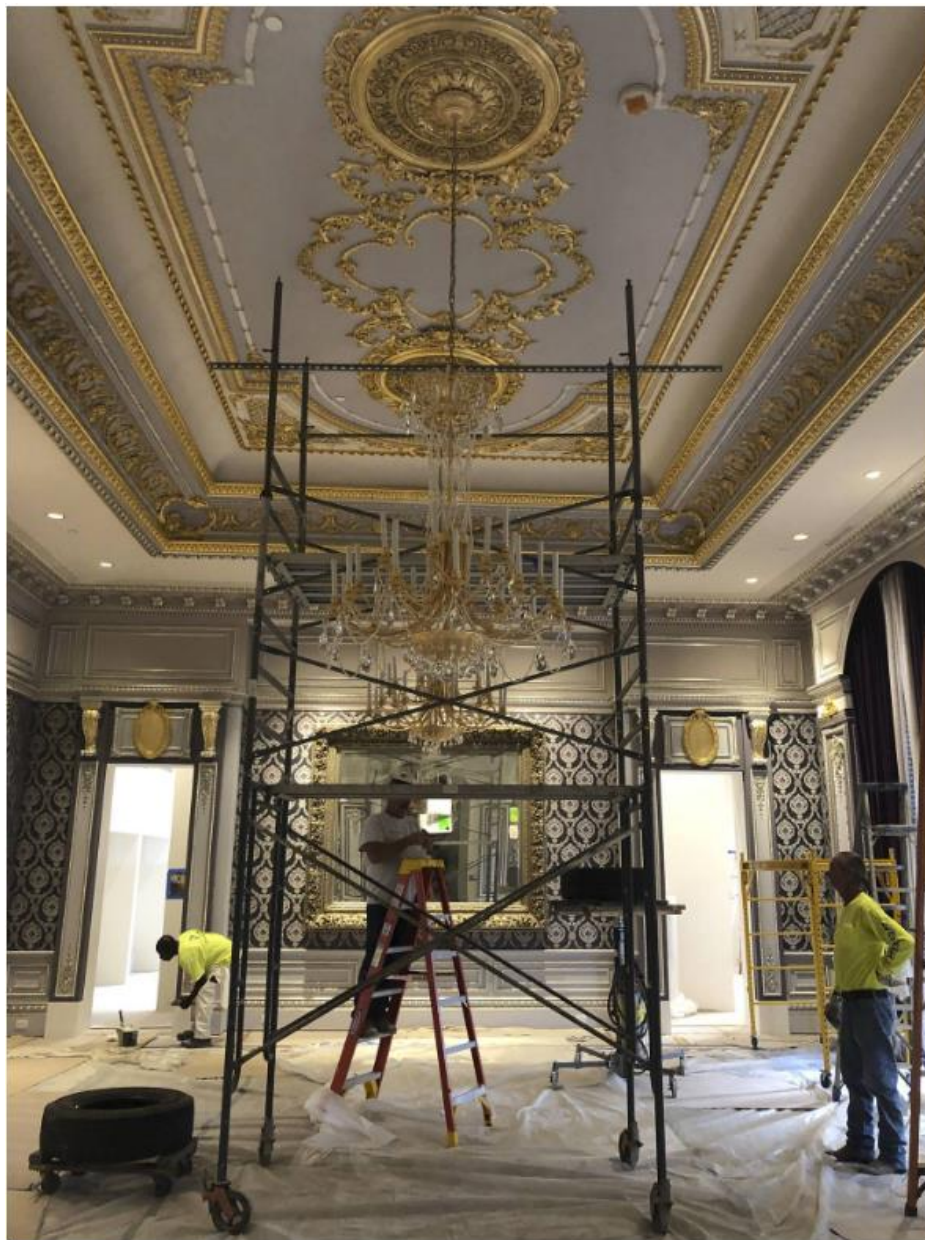
Construction on one of the dining rooms inside Versailles. (Courtesy photo)
